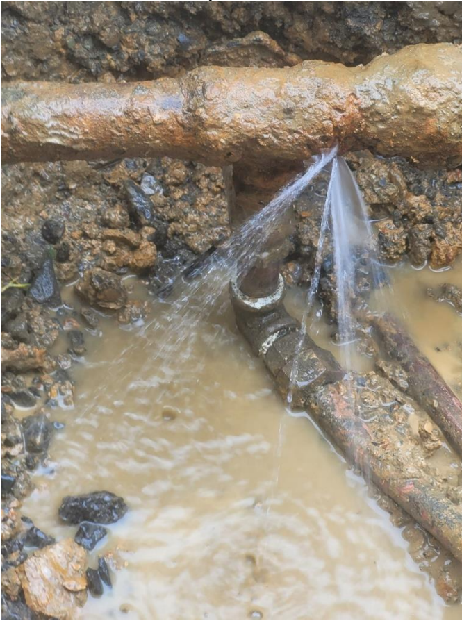
Noble Avenue water repair
