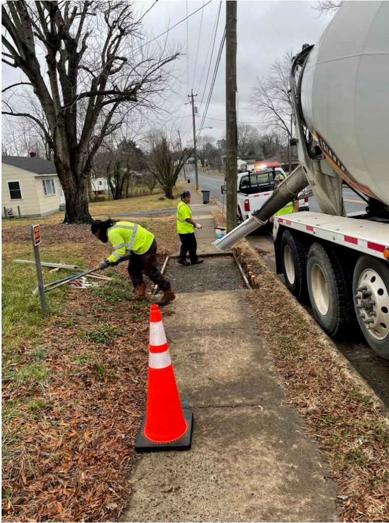
High Street sidewalk repair
